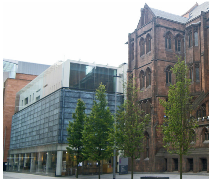
The John Rylands Library shows how new buildings (left) can complement historic ones.
