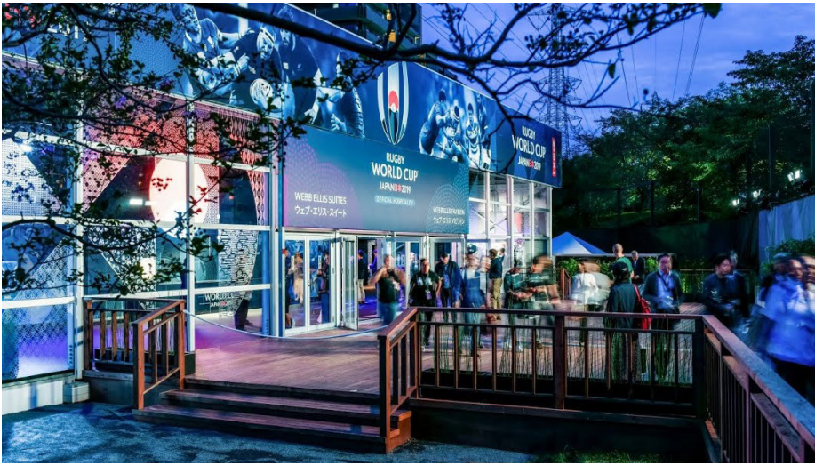
The Webb Ellis Pavilion in Yokohama built for the 2019 Rugby World Cup
