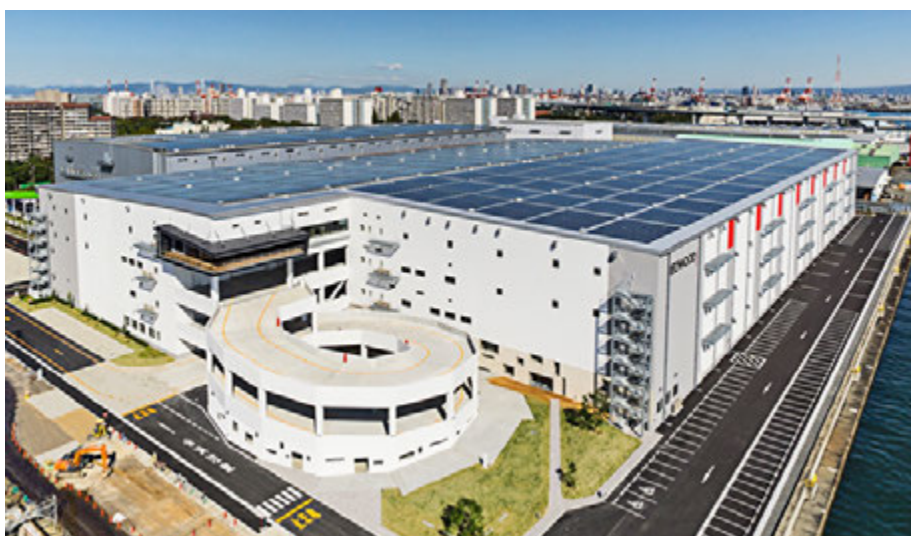
All ESR facilities have solar panels.
