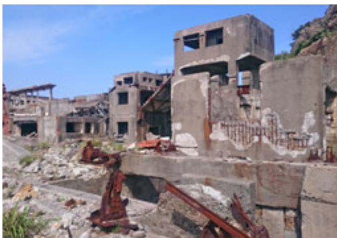
Much of the island is in severe decay. • PHOTO BY PETER TASKER
