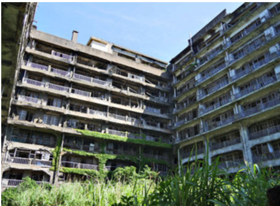
Many of the buildings have been taken over by nature. • PHOTO: GUNKANJIMA CONCIERGE
