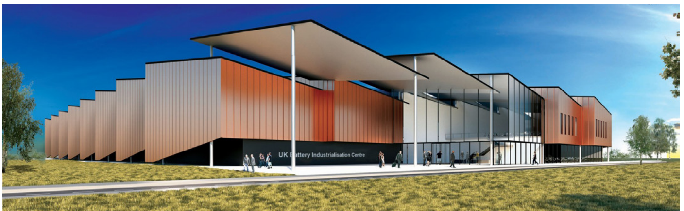
UK Battery Industrialisation Centre near Coventry
